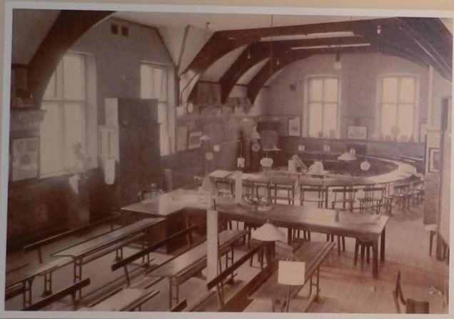
The new art room built in 1899. The curriculum from the 1840s onwards was very limited, concentrating on Latin, maths and English grammar. In 1878 the range of subjects was expanded to include French, natural science and drawing. Entrance exams were also introduced.
