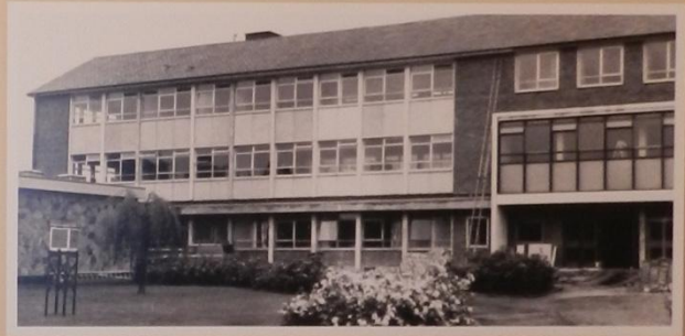
The building of the new school on Chatsworth Road was done in phases. The first phase included the science and maths block and was completed in 1961. These classrooms were used by the school while the second phase was completed.
